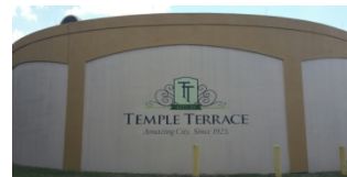
1 M.G. Water Storage Tank
